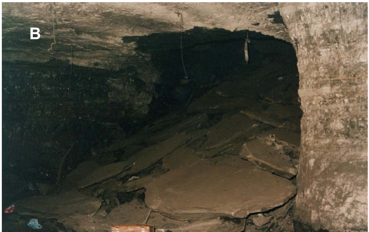
Figure 11 A & B – Roofbolts acting as a caving breakerline in A and no breakerline at all in B, (Madden, 1989)
