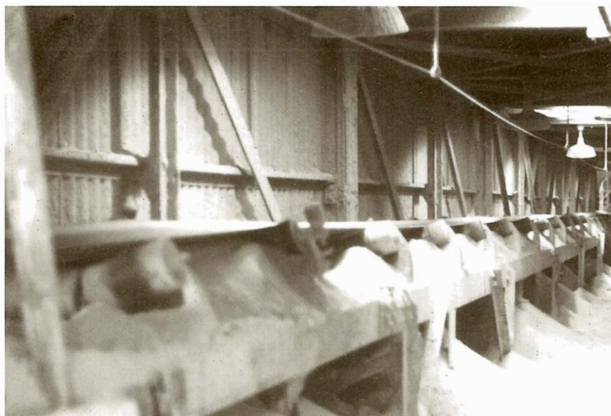
Inspection and action of system faults can prevent costly wear of the belt and idlers
